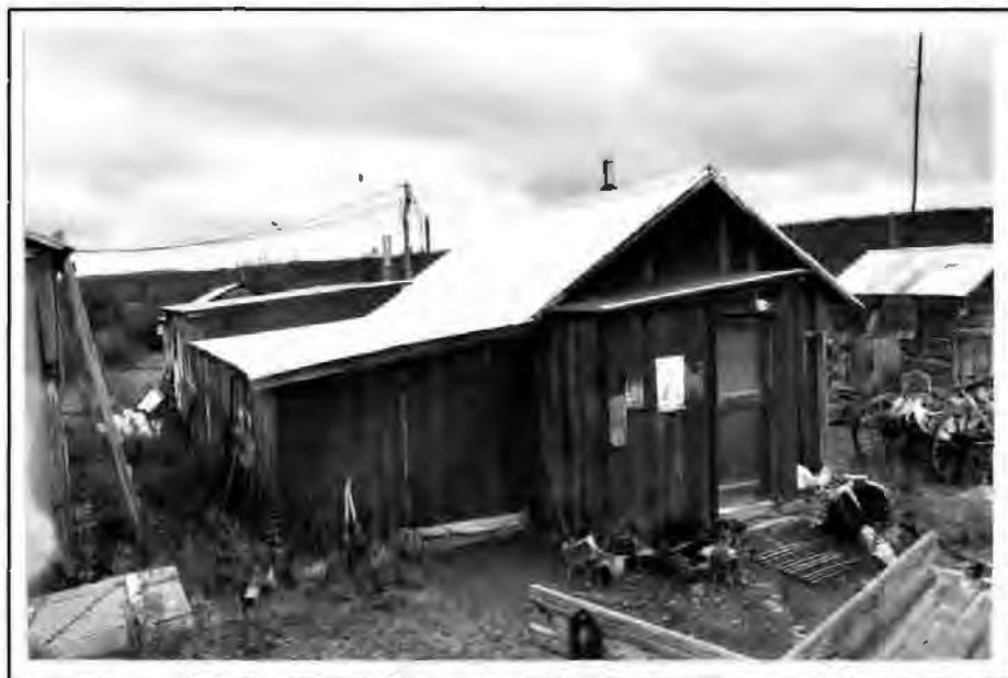
Figure 141. The Office and Workshop Building, 1993. The view is looking southeast.
